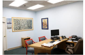
Big Shine Energy designed a layout that eliminated 21 unnecessary fixtures while increasing the light output from 30fc to 85fc.
