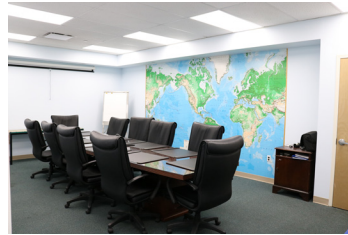
Big Shine Energy designed a layout that eliminated 21 unnecessary fixtures while increasing the light output from 30fc to 85fc.
