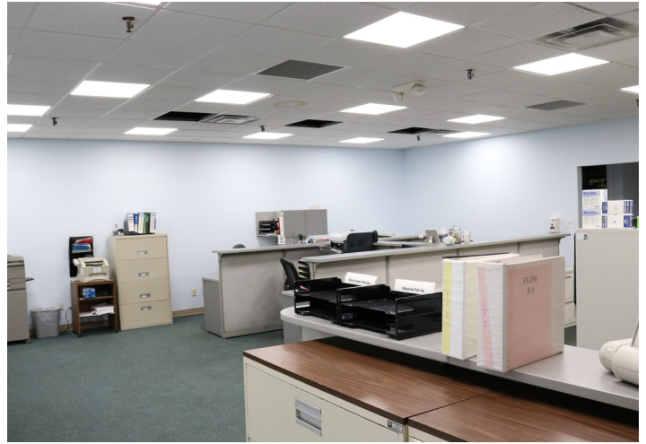
Big Shine Energy designed a layout that eliminated 21 unnecessary fixtures while increasing the light output from 30fc to 85fc.
