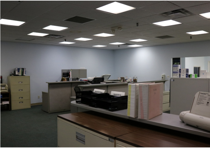
Wolf X-Ray's existing lighting layout was consuming significant amounts of energy while only producing minimal lighting.
