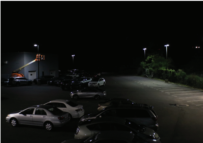
Existing metal halide fixtures left the A1's parking lot dim with minimal footcandle presence.
